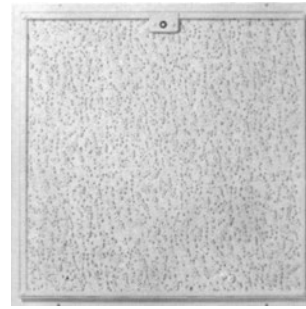
Finished inspection hatch
